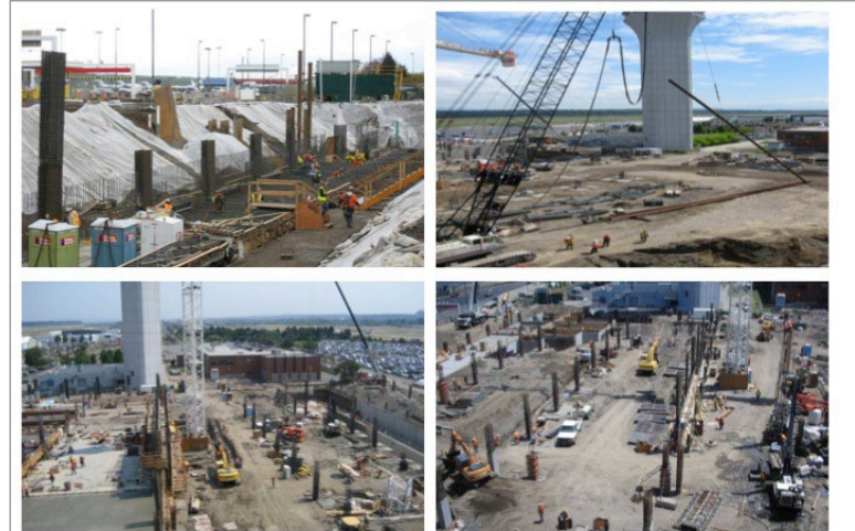
Passenger & Utility Tunnel Construction & Foundations - over 1,600ea. 120' long steel piles
