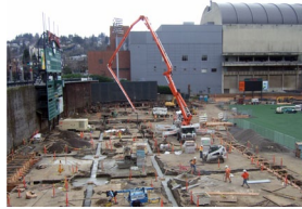
March 2010 Phase 1 Foundations Laid
